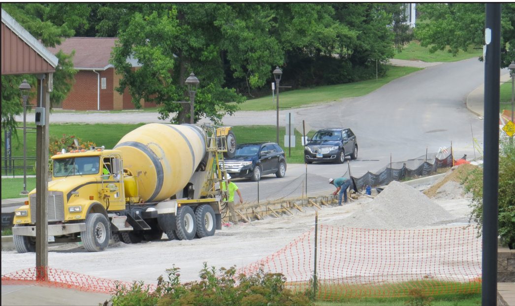
A new parking lot is under construction on the site of a former playground at the city park.
