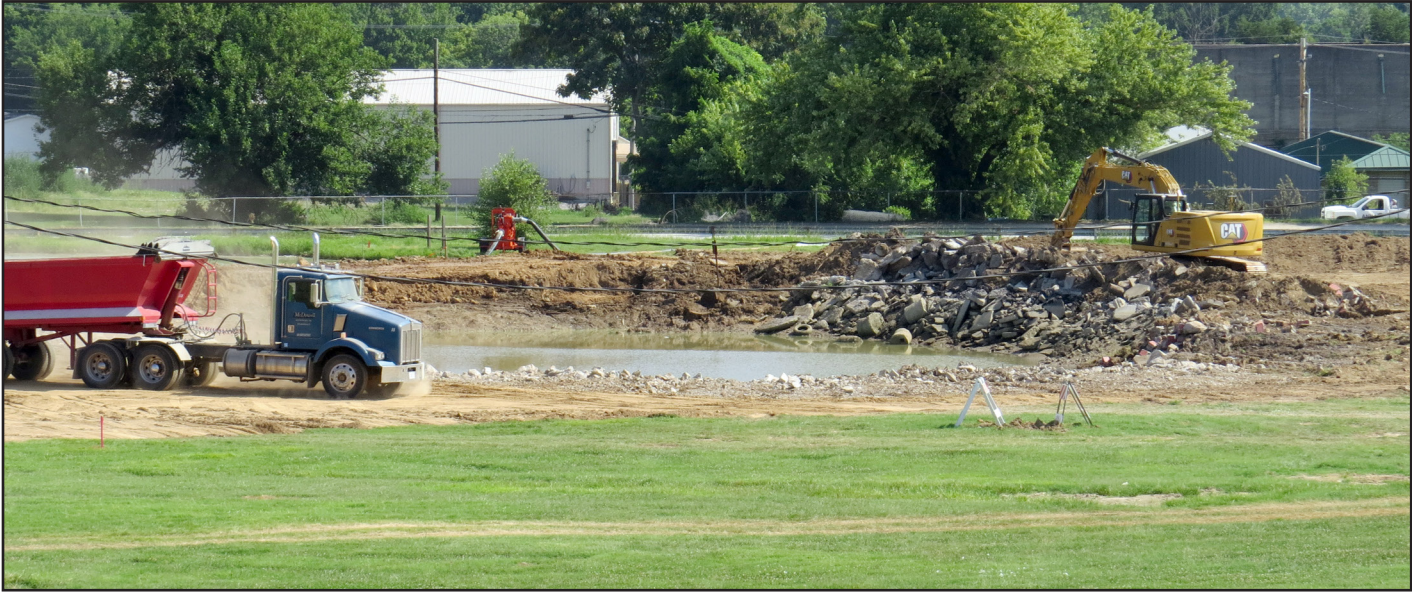
Park project brings changes to pond A major improvement project which is underway is bringing some big changes to a pond at the Anna City Park. The accompanying photographs were taken while work was being last week at the park. Dirt was being dropped by a truck along the edge of the pond on July 23. The water level in part of the pond had dropped when another photograph was taken July 25.
