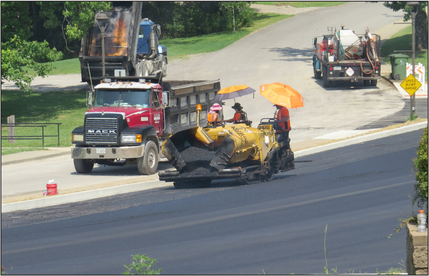
Parking lot project progress One of a number of improvements which can be seen at the Anna City Park is a new parking lot. The parking lot is located at the site of a former playground. Paving work was followed last week by the painting of stripes on the new lot.
